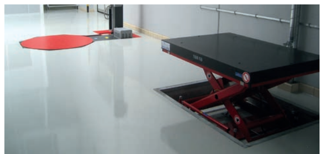
Conductive WHG coating in a production hall
