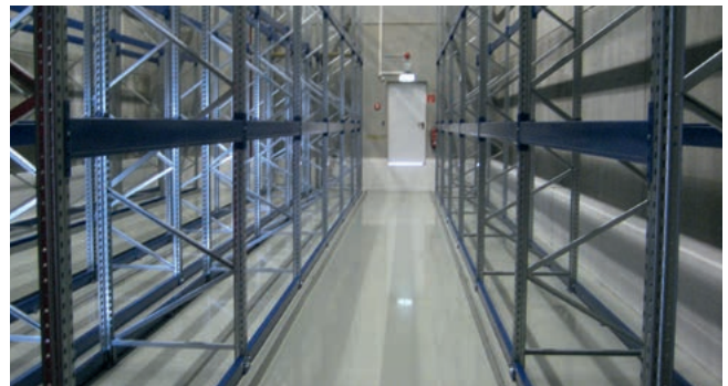
WHG coating in a shelf storage warehouse
