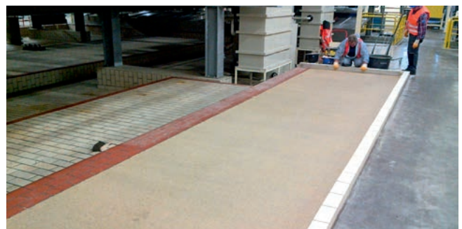
Installing a screed coating
