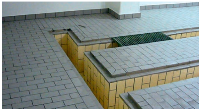
Combined covering implemented with gutters
