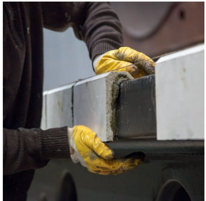
Working with synthetic resin mortar
